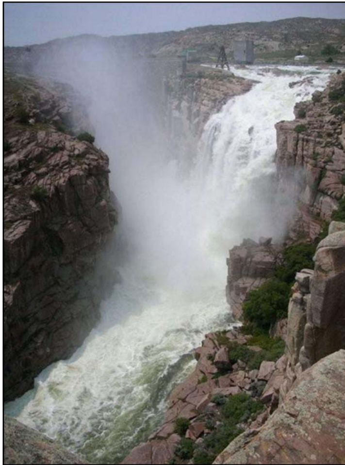
The spillway at Pathfinder Dam, southwest of Casper, Wyoming, ran for several days in June 2010, the first time since 1984. (Photo courtesy of The Central Nebraska Public Power and Irrigation District.)
