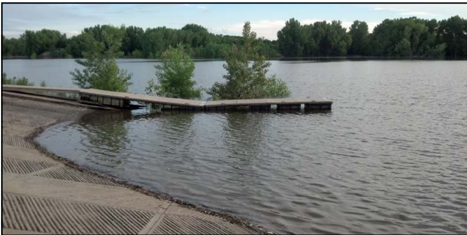
Elwood Reservoir in June 2015.
