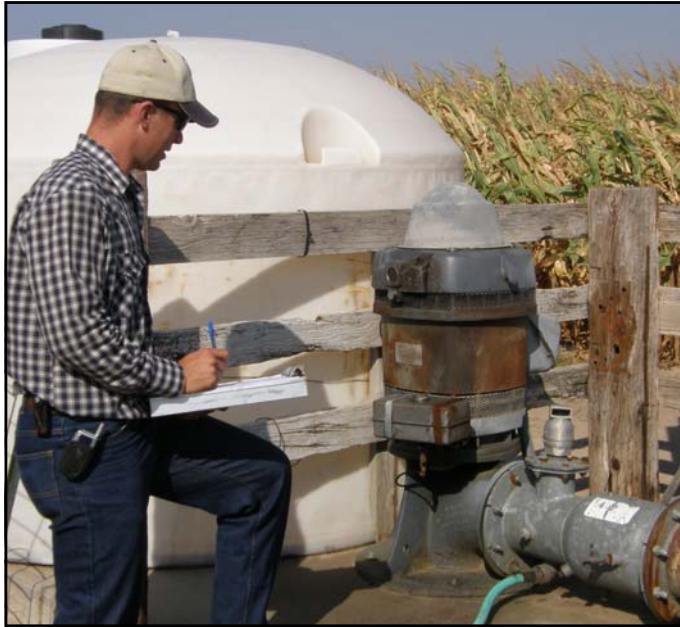
TBNRD Water Resources Manager Nolan Little inspects a chemigation system.
